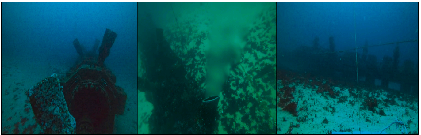
Fig. 4. Brine discharge outfall from Candelaria desalination plant.
