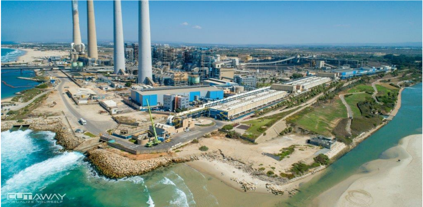
Figure 3: Near Shore Discharge - Hadera Desalination Plant
